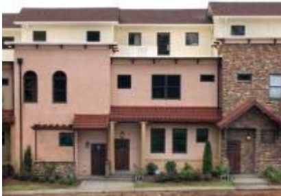
The townhouse units at Camp Creek Village are designed to resemble Mediterranean villas.
